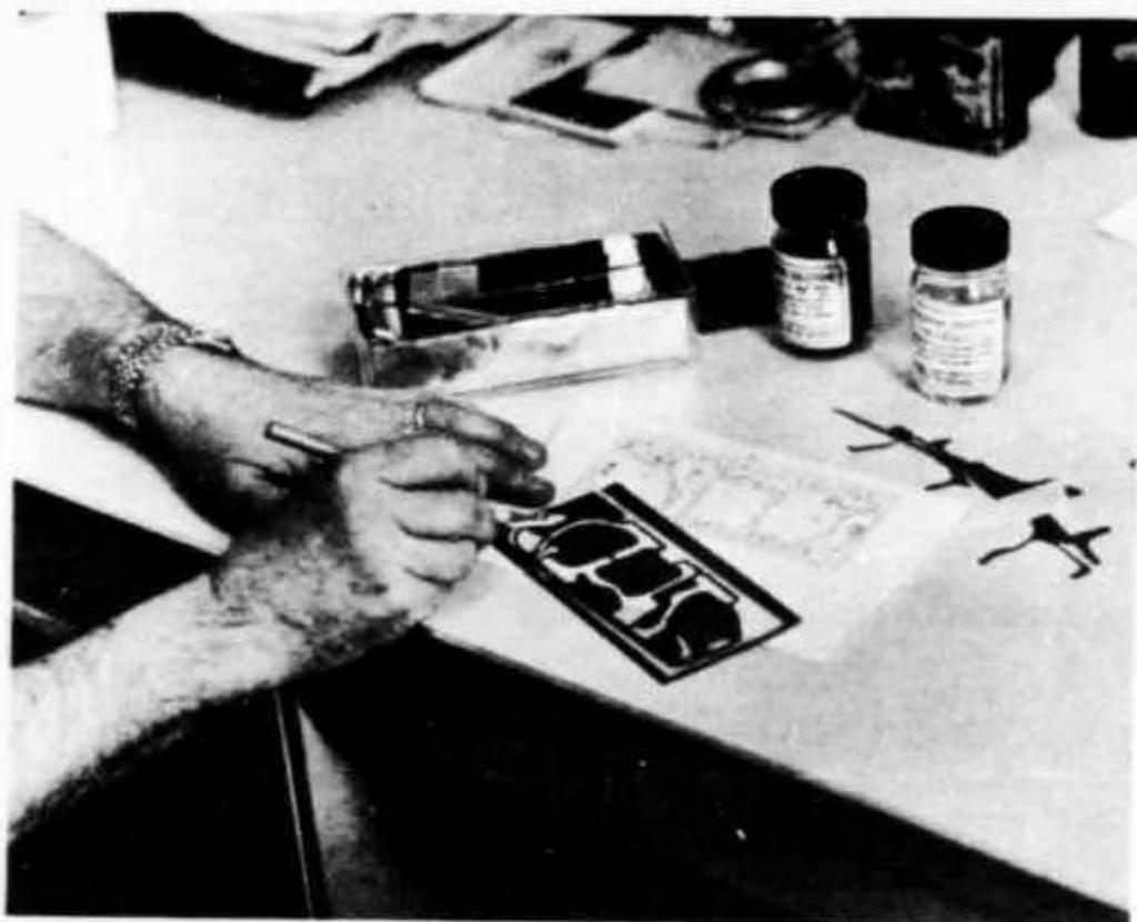
In this photo a negative of the circuit-board pattern is being prepared by cutting away the unwanted sections with an X-acto knife. The pattern on the negative is the same as that of the original drawing shown adjacent to it. This negative is for use during photo-etching, and is part of a Kepro kit.
