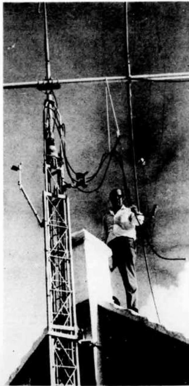
Ed Kelly, VP9GE, examines the driven element of the four-element quad before it is cranked to contest height.
